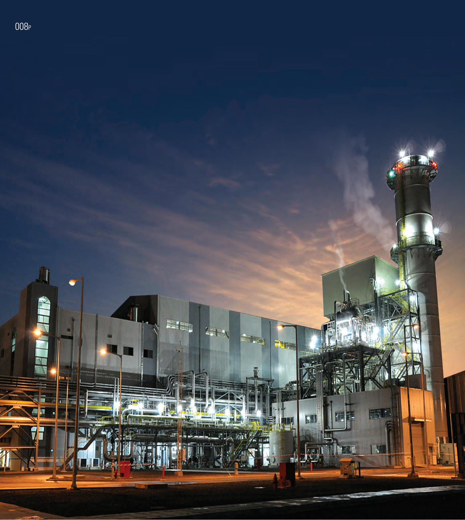
008P Yerevan Combined Cycle Power Plant Location: Yerevan, Armenia - Total 230MW - Gas Turbine 167MW×1 - Steam Turbine 63MW×1 Project period: 2007. 12 ~ 2010. 04
