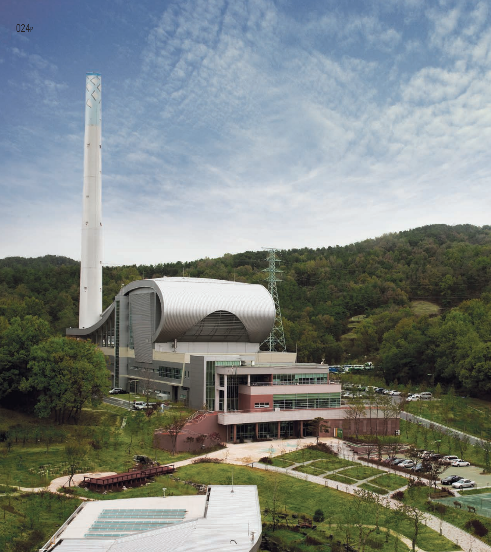
024P Cheongju Municipal Solid Waste Treatment Plant
